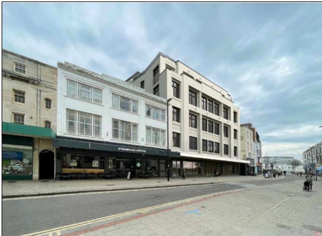
Figure I. View of proposed frontage of the building.
